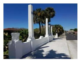
The rehabilitation of the National Register of Historic Places-eligible Main Street Bridge over Hogans Creek served as a unique solution to a structurally deficient bridge. Constructed in 1929, the Main Street Bridge existed as a single span reinforced concrete slab structure and functioned as a four lane roadway with a sidewalk along each outside travel lane for vehicles and pedestrians traveling between the Historic Springfield neighborhood and downtown Jacksonville.
